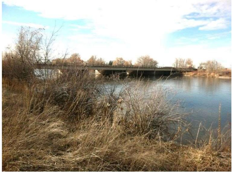
Design requirements and design capacity of bridges across the River in the study area were not reviewed. The FEMA flood insurance study profiles indicate the SH-26 Bridge should pass the FEMA predicted 100-year water elevations approximately 0.5 feet under the low chord of the bridge, including the FEMA estimated effects of ice jams.
